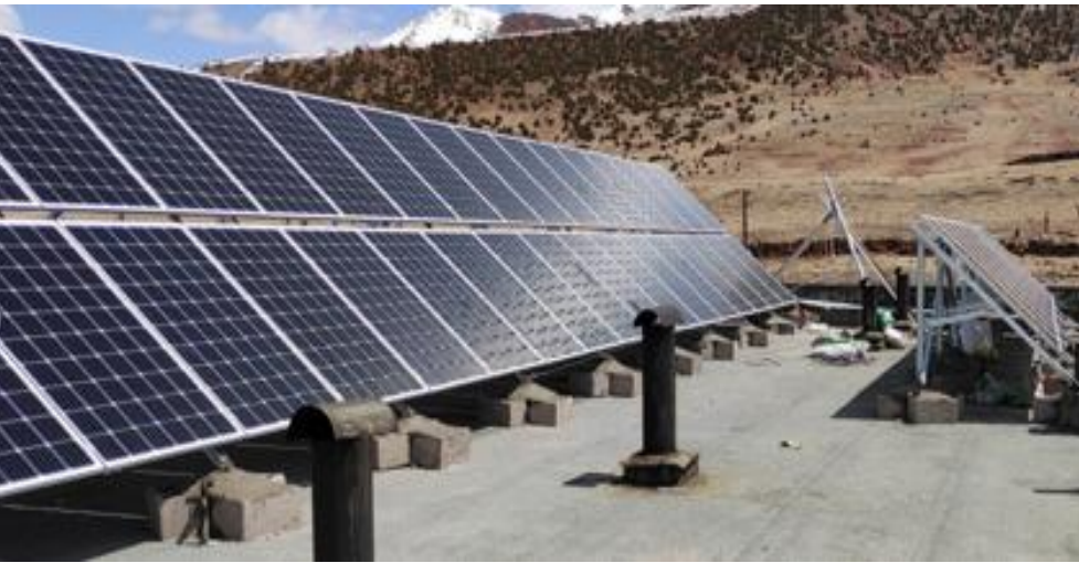
Yushu 30kW photovoltaic off-grid
